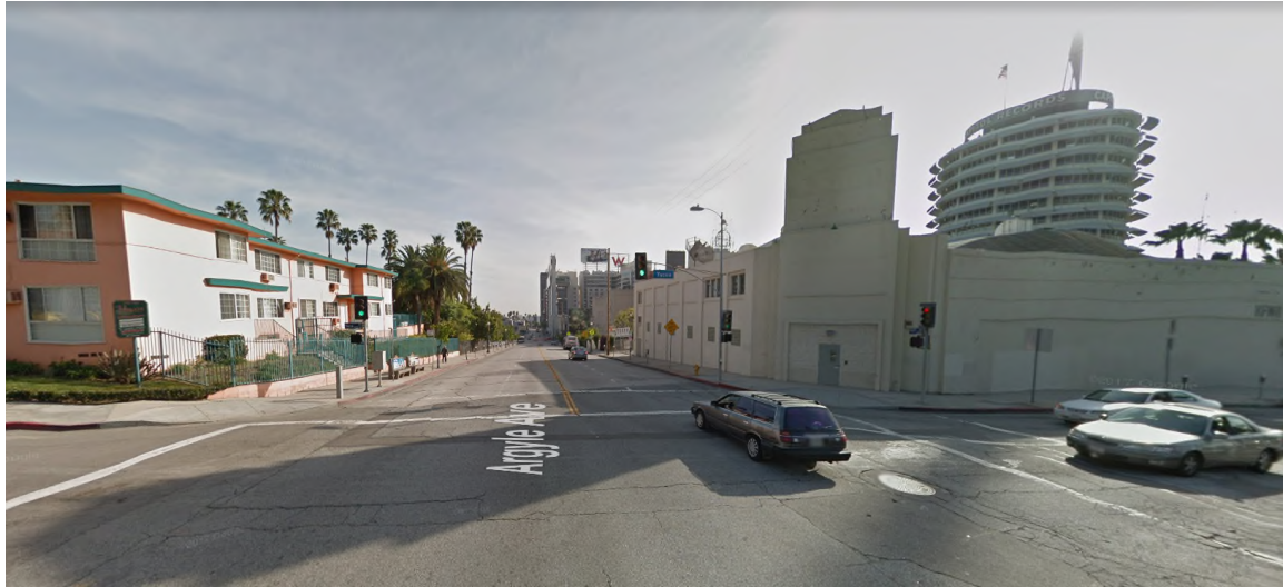
4. Yucca Street and Argyle Avenue, facing south
